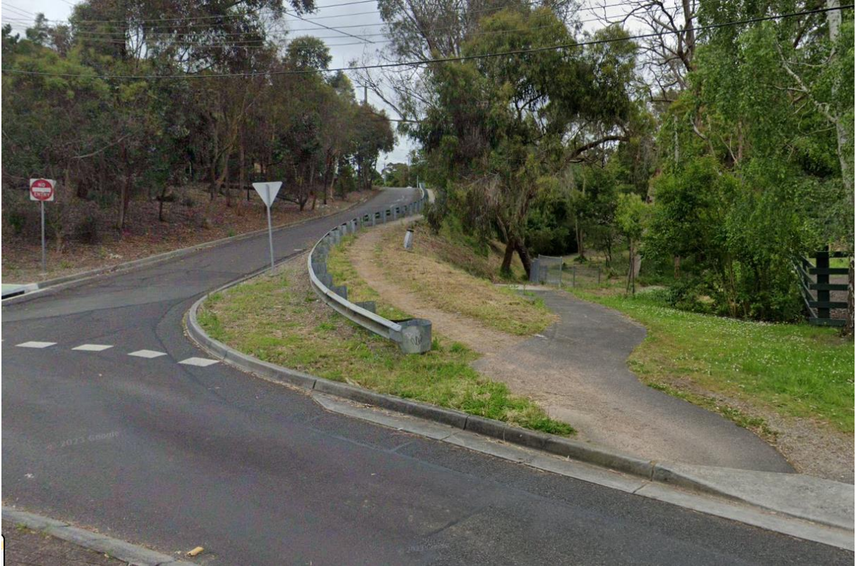
Existing trail along Maroondah Hwy at Birts Hill
